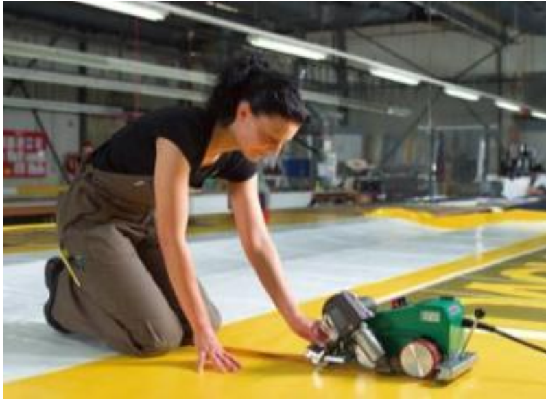
Hot-air welding machine (Uniplan) driving over laid-out truck covers
